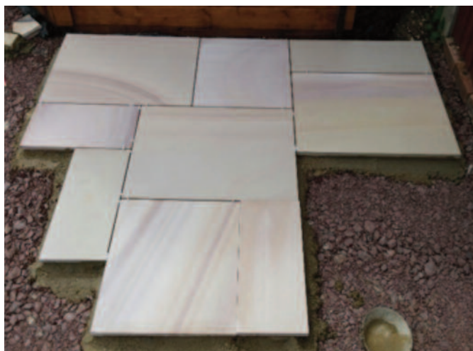
Spacers not advised. Minimum 2mm joint.
